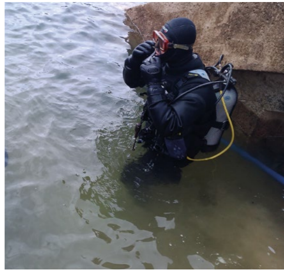
Underwater installation of sensors in Mavrovo Dam
