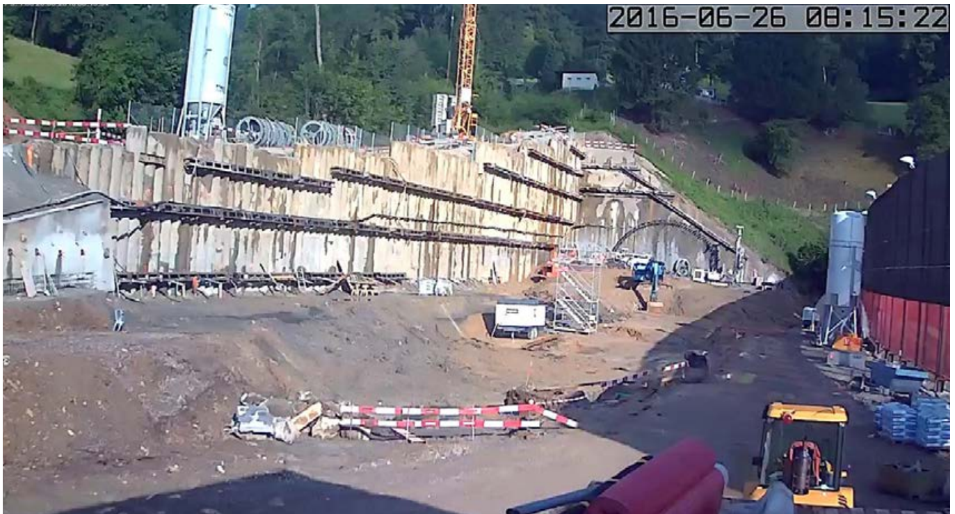
Webcam-picture of retaining wall
