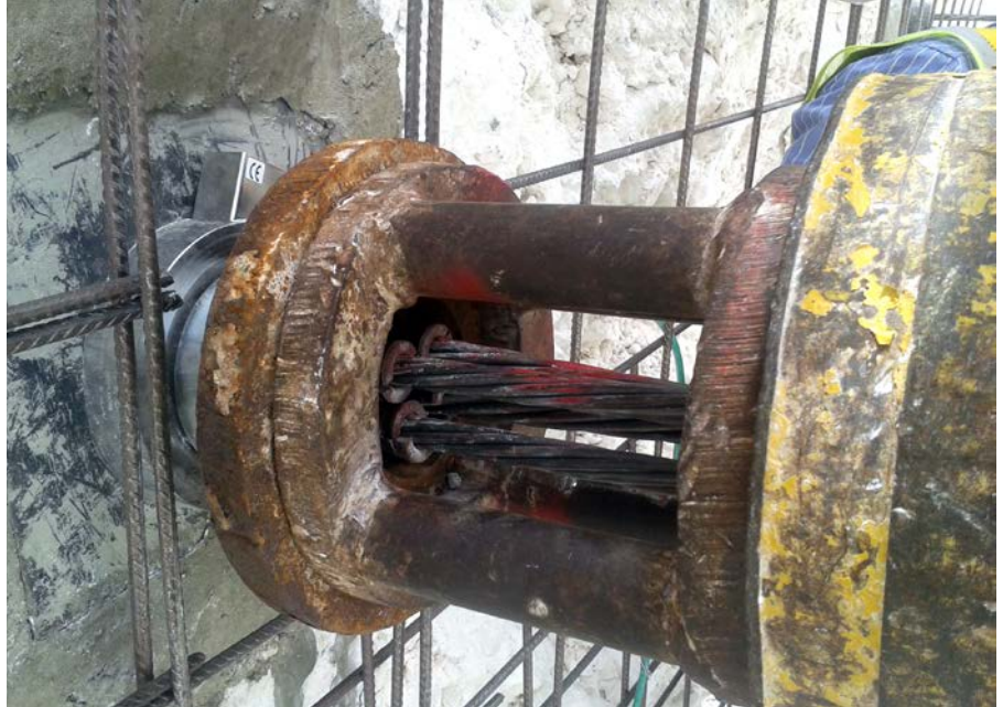
Anchor tensioning with the installed anchor load cell
