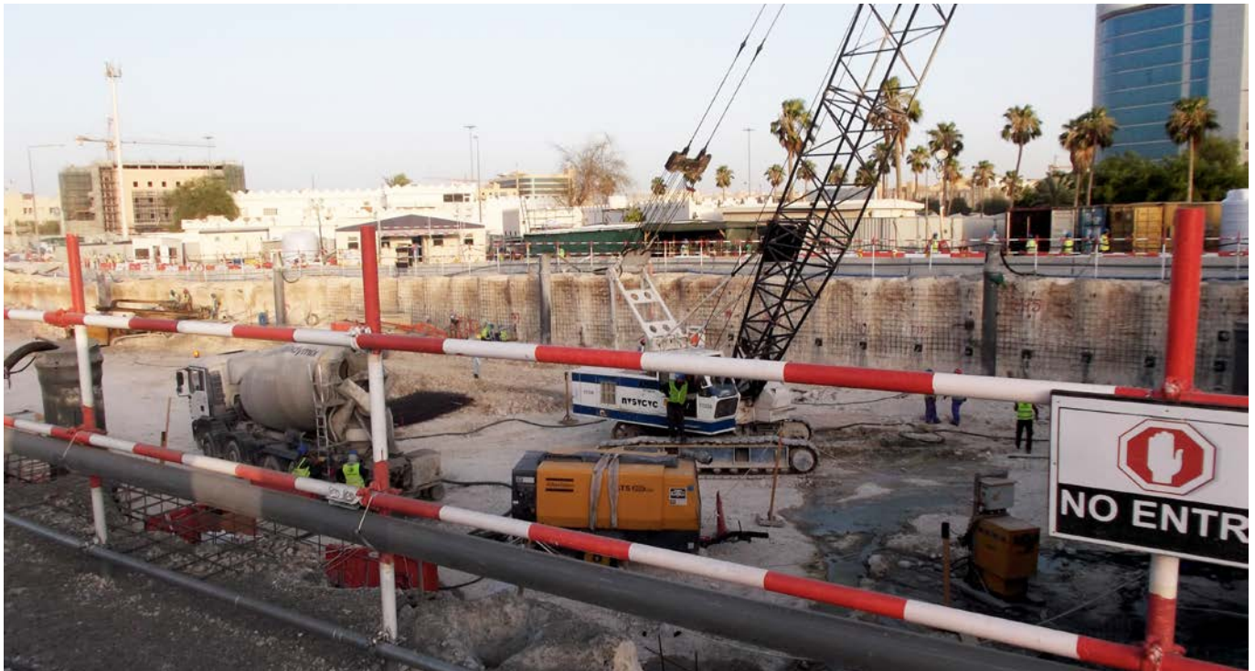
Excavation, just started, with first row of anchors
