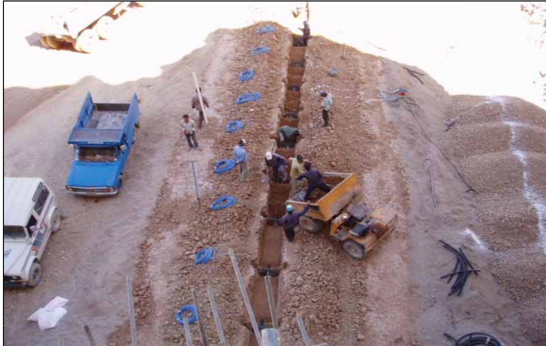
Installation of embankment extensometers
