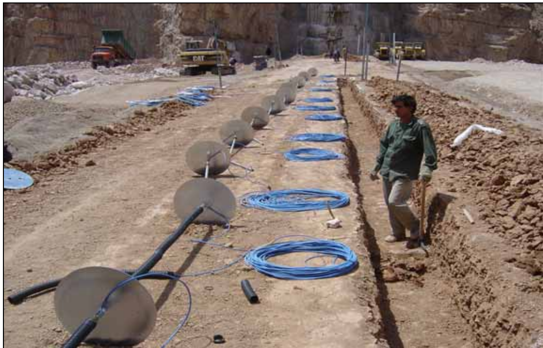
Trench for installation of embankment extensometers
