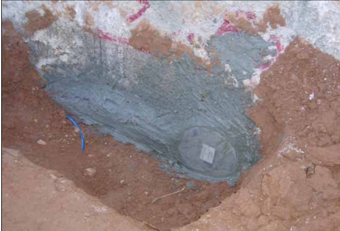
Installation of earth pressure cell
