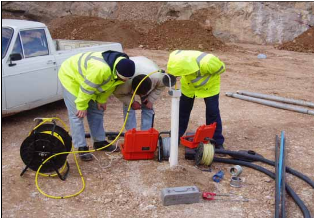
Vertical inclinometer measurements
