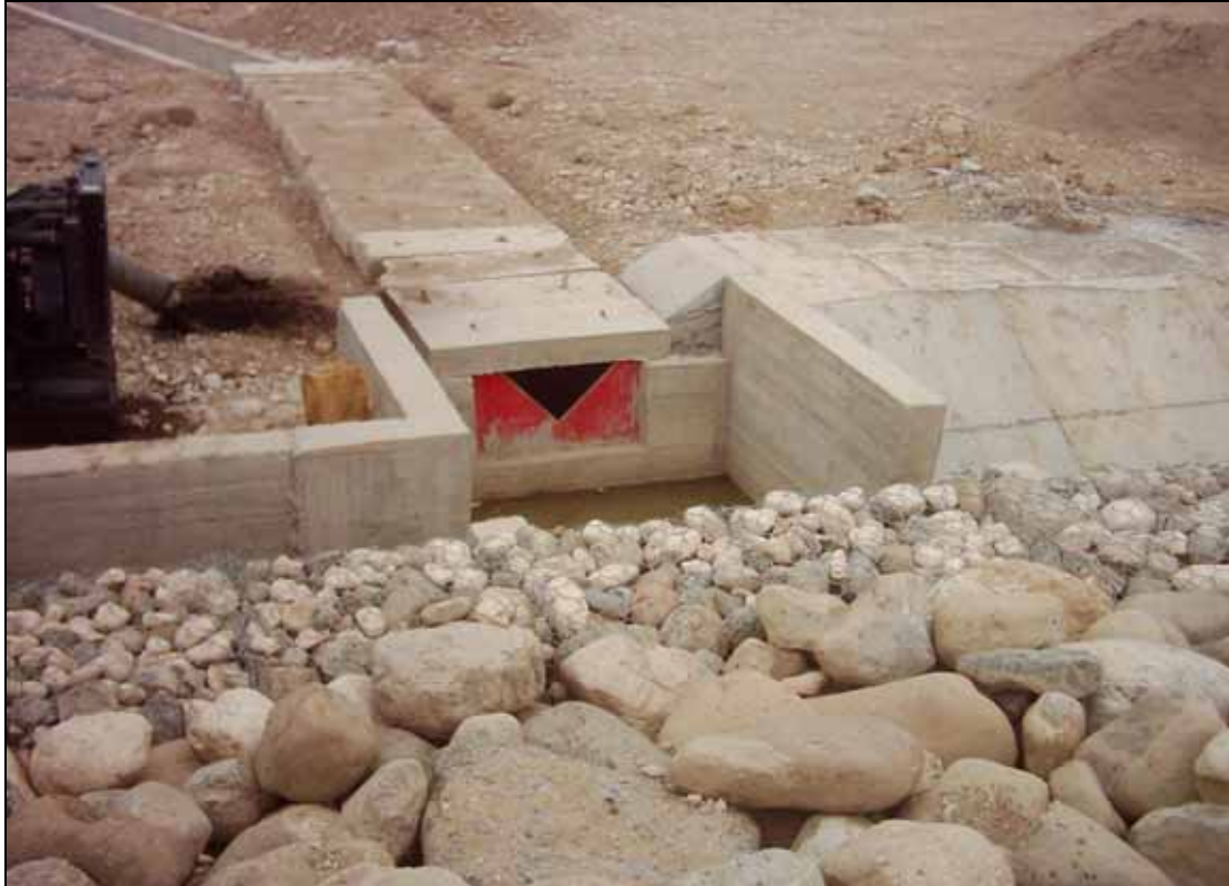
V-notch on dam downstream for leakage measurements
