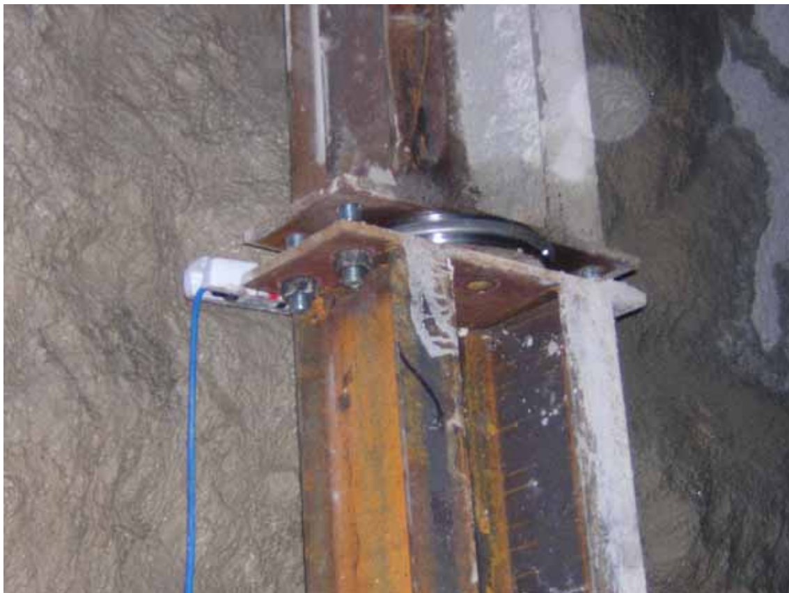
Steel lining load cell installed between two section of linings
