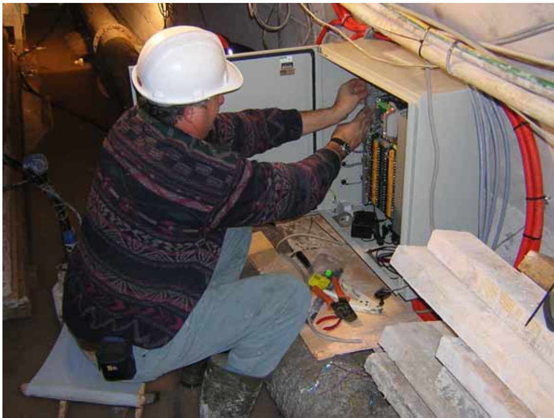
Wiring procedures on the ADK-10 data acquisition system
