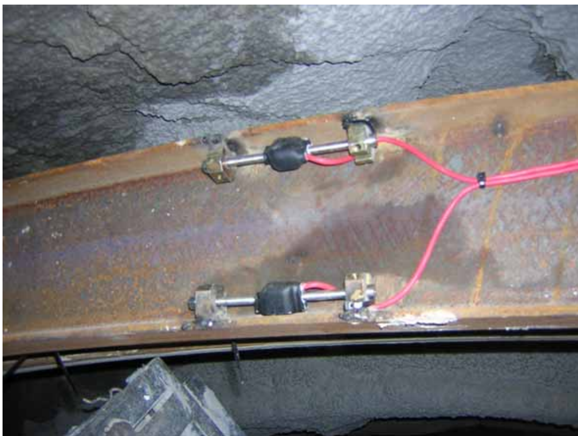
Vibrating wire strain gauges installed on steel lining
