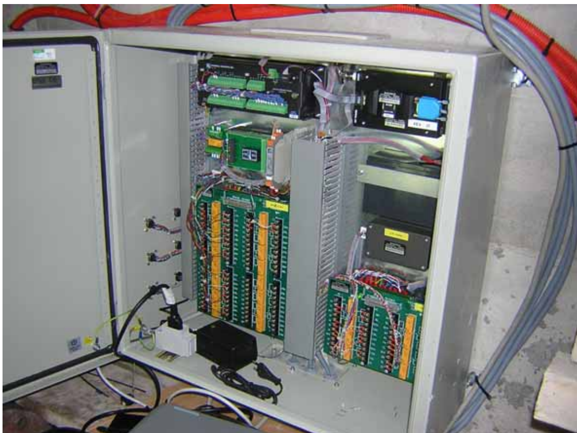
ADK-10 automatic data acquisition system
