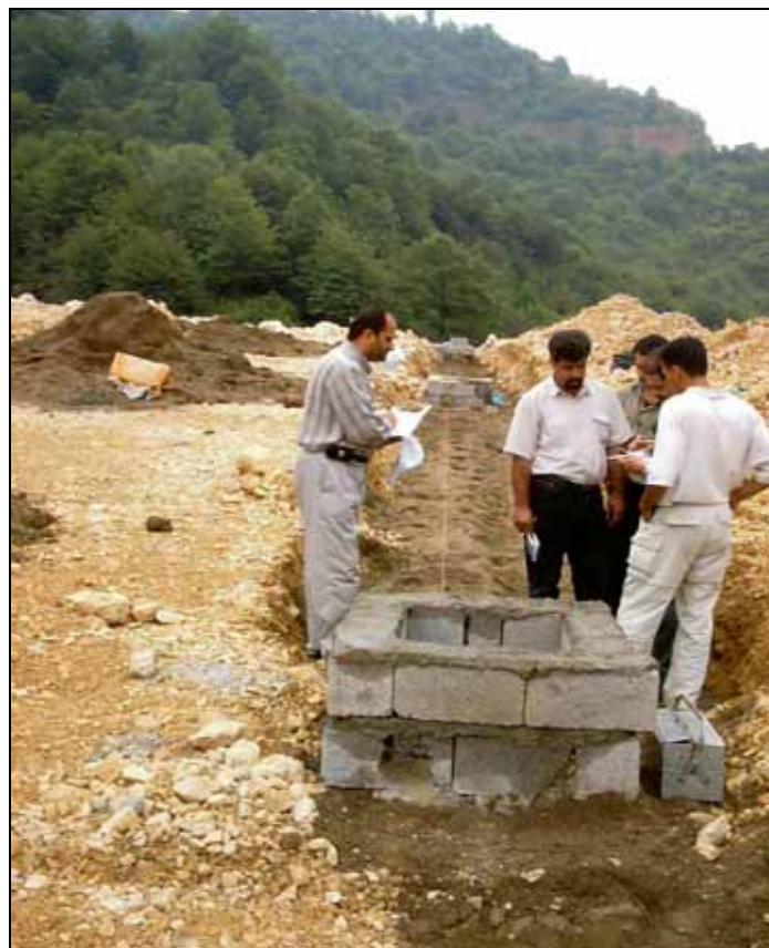
Installation of DSM hydraulic settlement system for embankment
