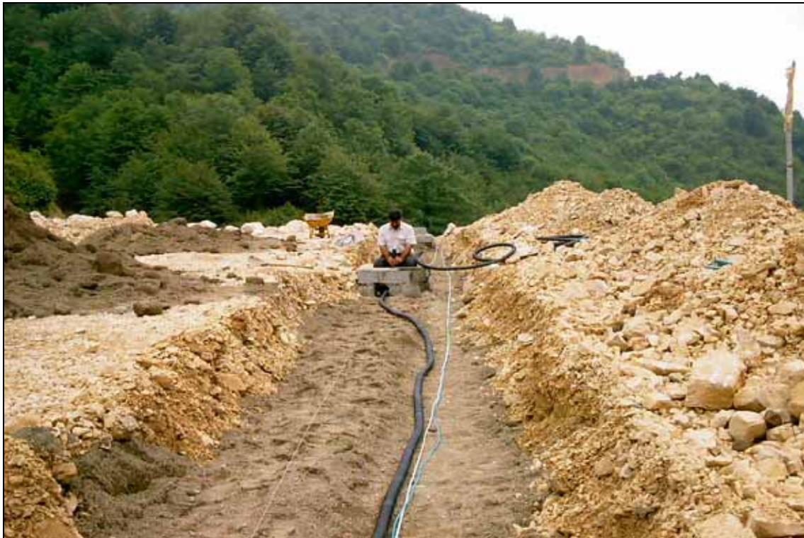
Installation of DSM hydraulic settlement system for embankment
