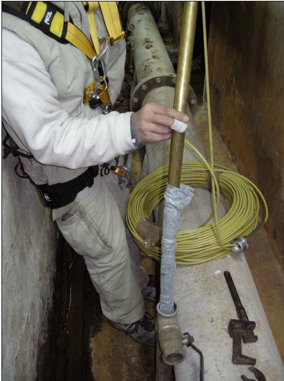
Installation of the pore pressure trasducer within the dam foundation
