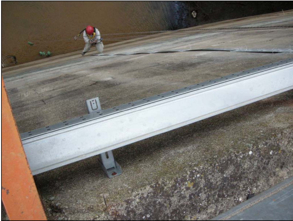
Installation of the hydrometric rod
