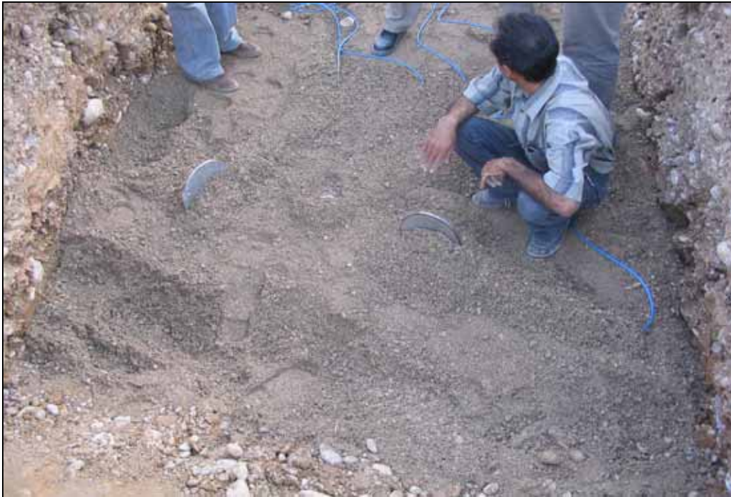
Installation of earth pressure cells
