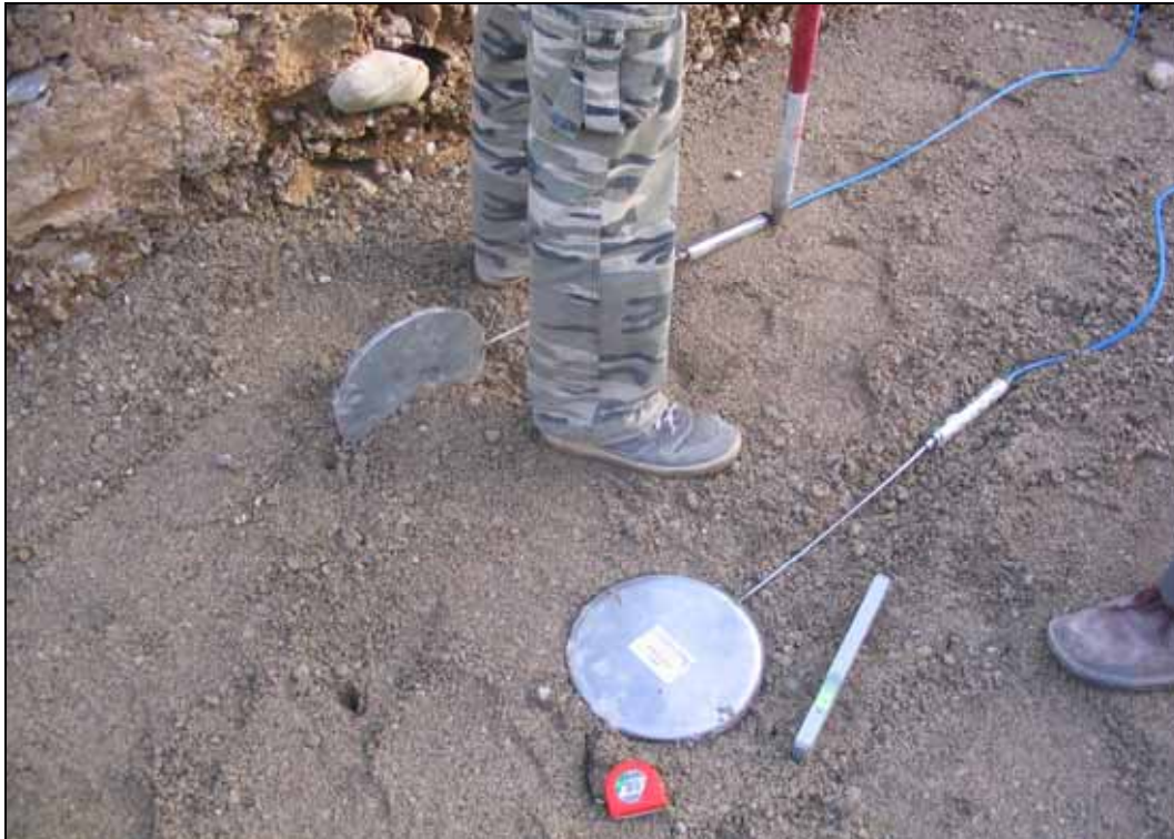
Installation of earth pressure cells in two directions
