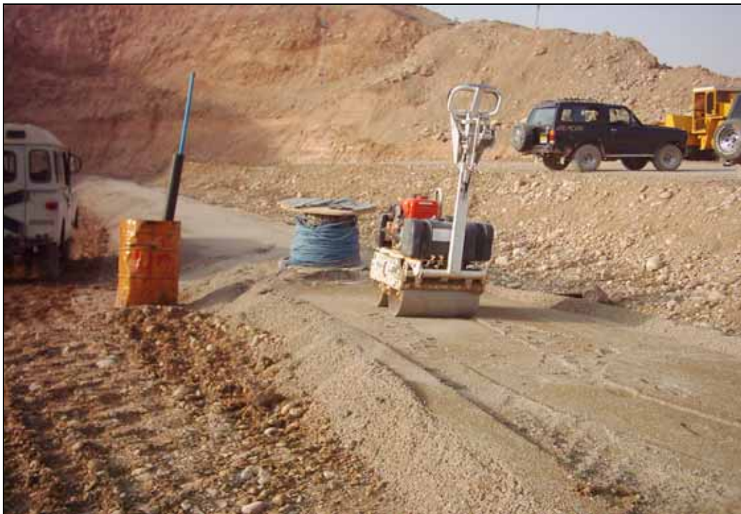
Compaction of sand after earth pressure cells positioning
