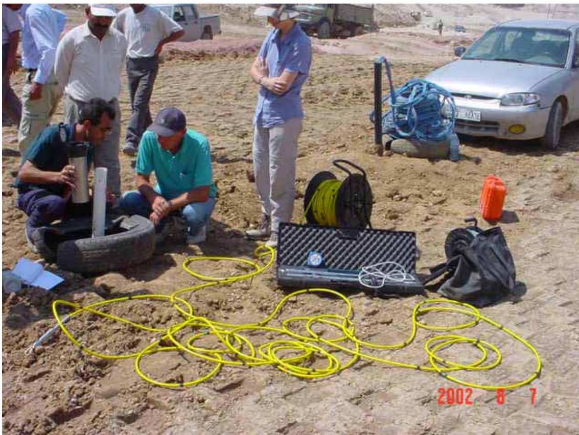
Inclinometer measurements during earth-fill embankment construction
