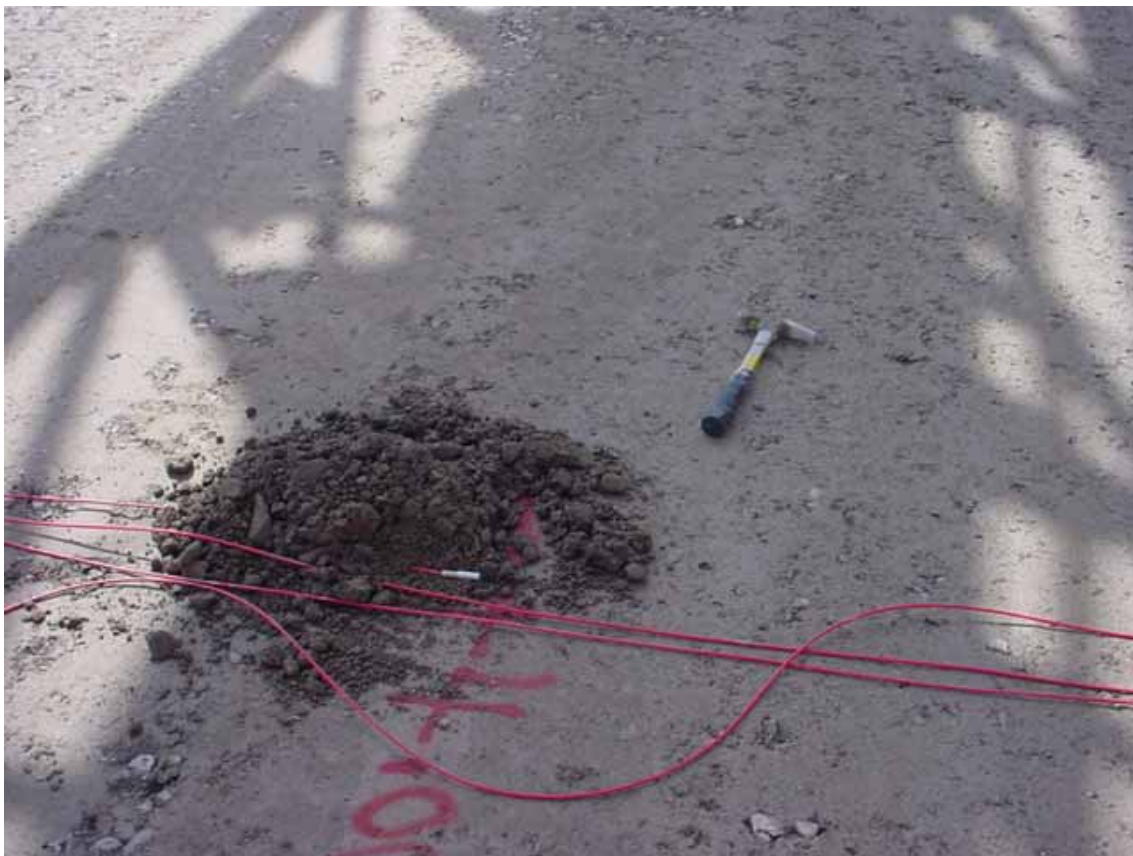
Installation of temperature gauge within RCC dam body
