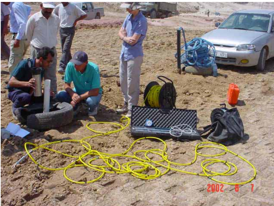
Inclinometer measurements during embankment construction
