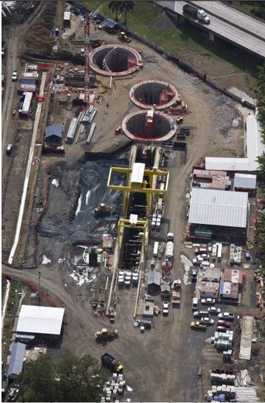
Chanis pumping station pits - May 2011
