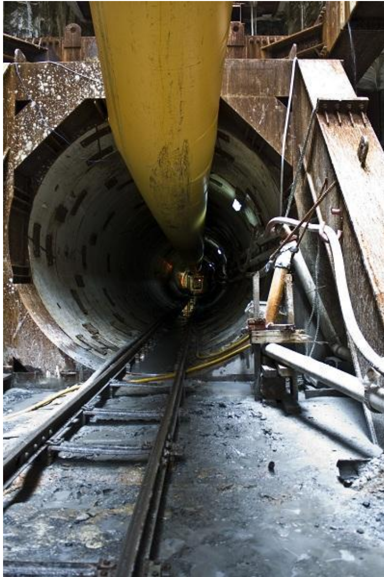
Panamá TBM EPB SBP Tunnel
