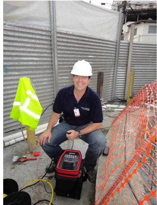
Inclinometer measurement at Pozo Santa Elena Panama City SBP
