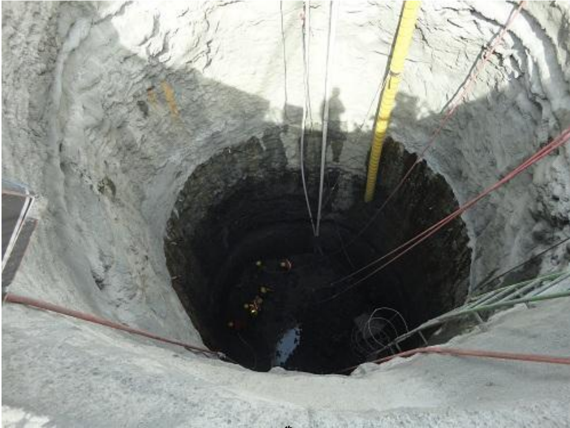
Pit of Santa Elena excavation – April 16 th 2011 - 2011 17,8 meter depth (approx.)
