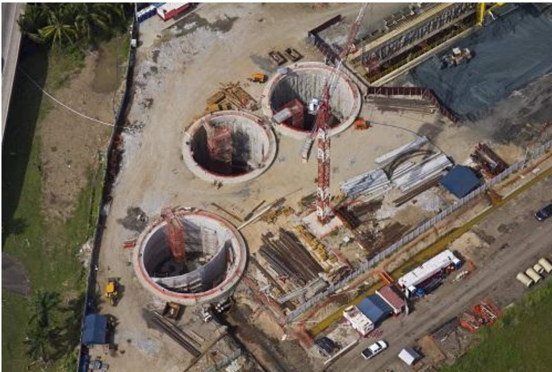
Pumping station - May 2011
