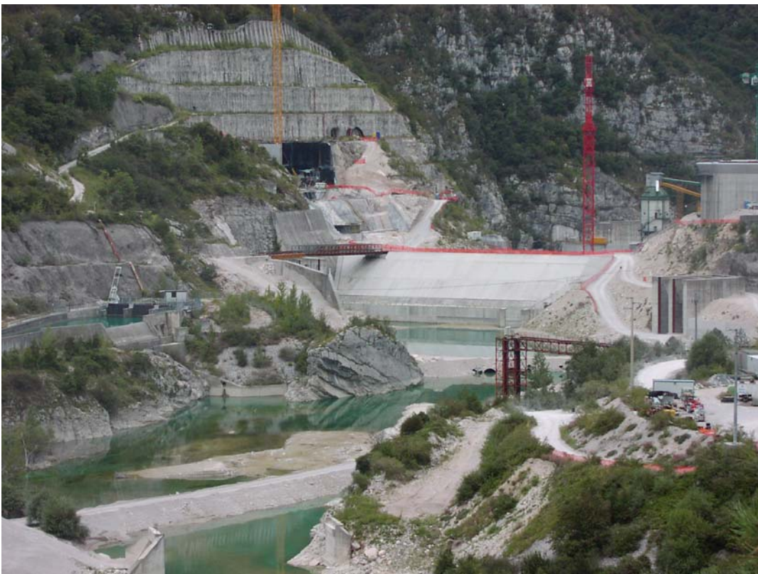
General view of the dam
