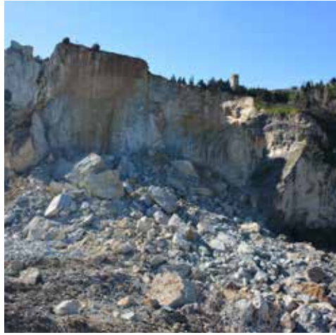
San Leo landslide monitoring, Italy
