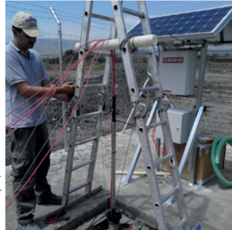
DEX-S inclino-extensometer installation, 150 mt depth, Ptolemaida Mine - Greece
