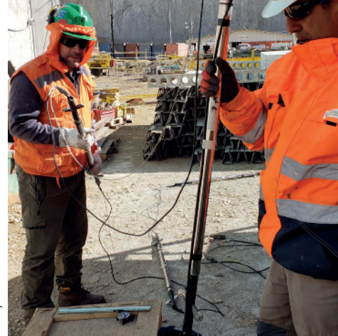
DEX-S inclino-extensometer installation, Chuquicamata Mine - Chile
