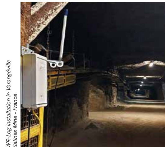
DEX-S inclinometer-extensometer installation, 150 mt depth, Ptolemaida Mine - Greece
