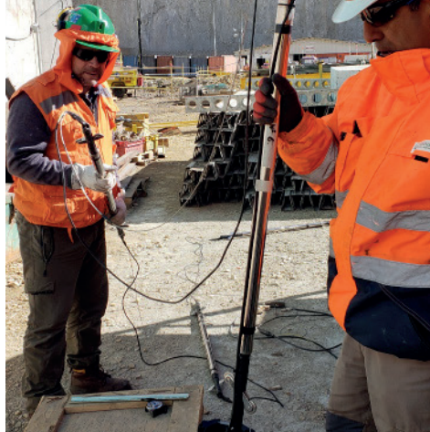
DEX-S inclino-extensometer installation, Chuquicamata Mine - Chile
