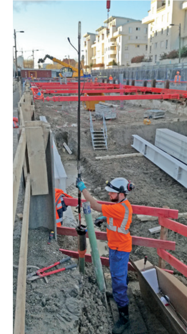
BH-Profile chain installation
