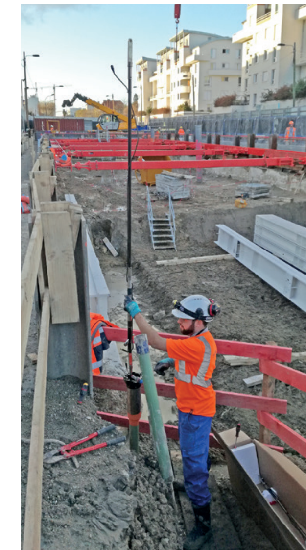
BH-Profile chain installation
