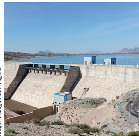
Ouladjet Mellegue dam, Algeria
