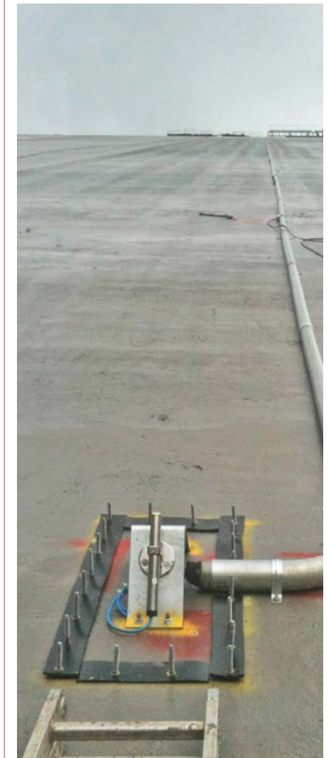
Submersible tilt meter installed on up-stream face of Sogamoso Dam - Colombia (190mt high)
