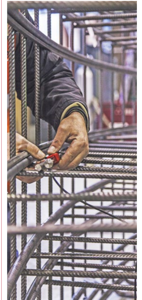
TELT - Tunnel Euralpin Lyon Turin, installation of VW strain gauges within TBM precast concrete element.
