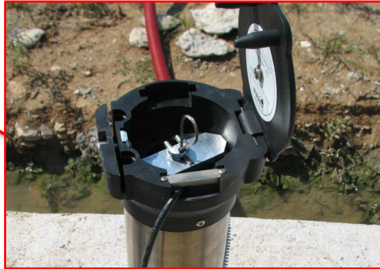
Support top cap after installation
