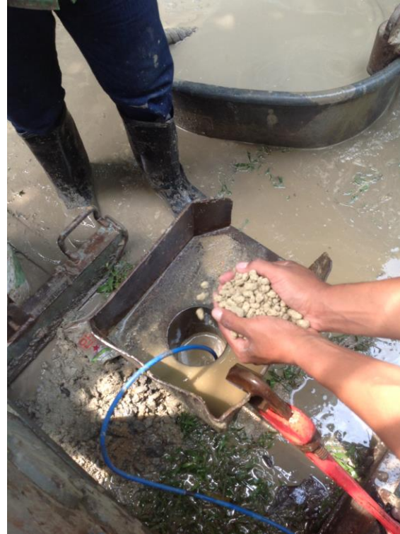
Filling with bentonite pellets (sealing)
