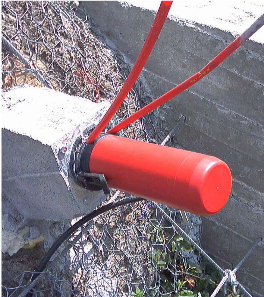
MPBX on dam abutment
