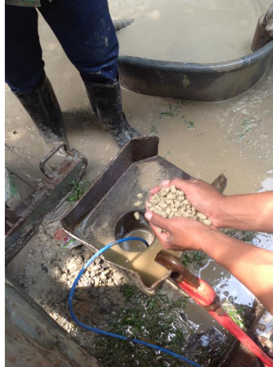
Filling with bentonite pellets (sealing)
