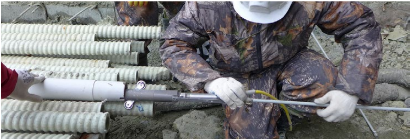
Preparing T-REX probe for horizontal surveying
