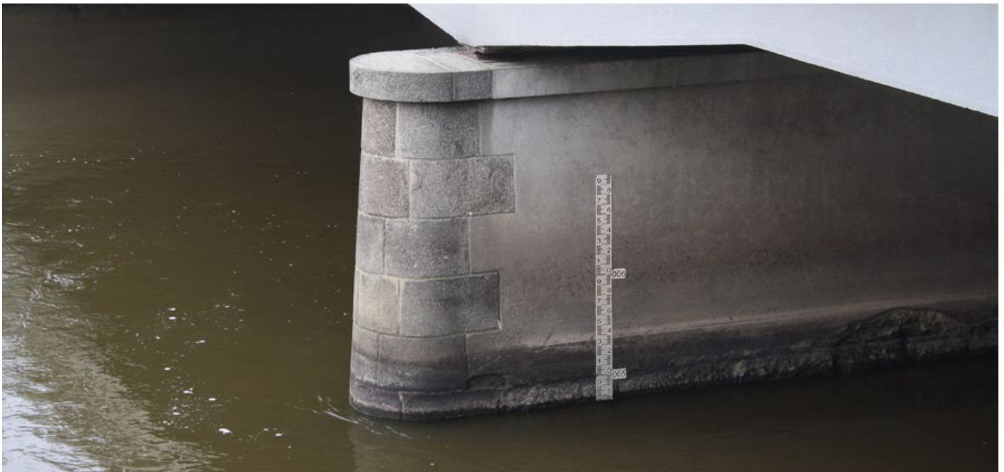
Staff gauges installed on bridge pillar
